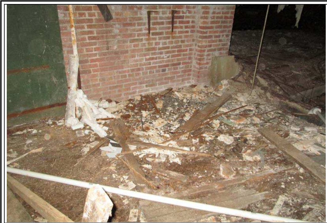
Photo 5 – View of Backstage Aircell Insulation Debris
