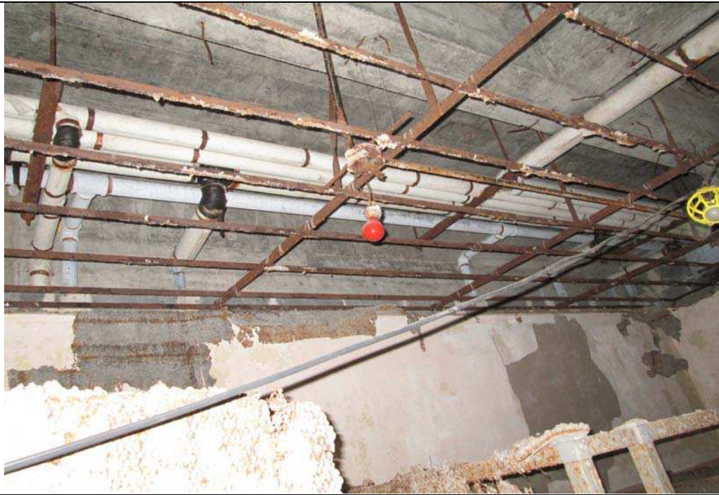
Photo 7 – View of Aircell Pipe Insulation in Women’s Bathroom in Basement
