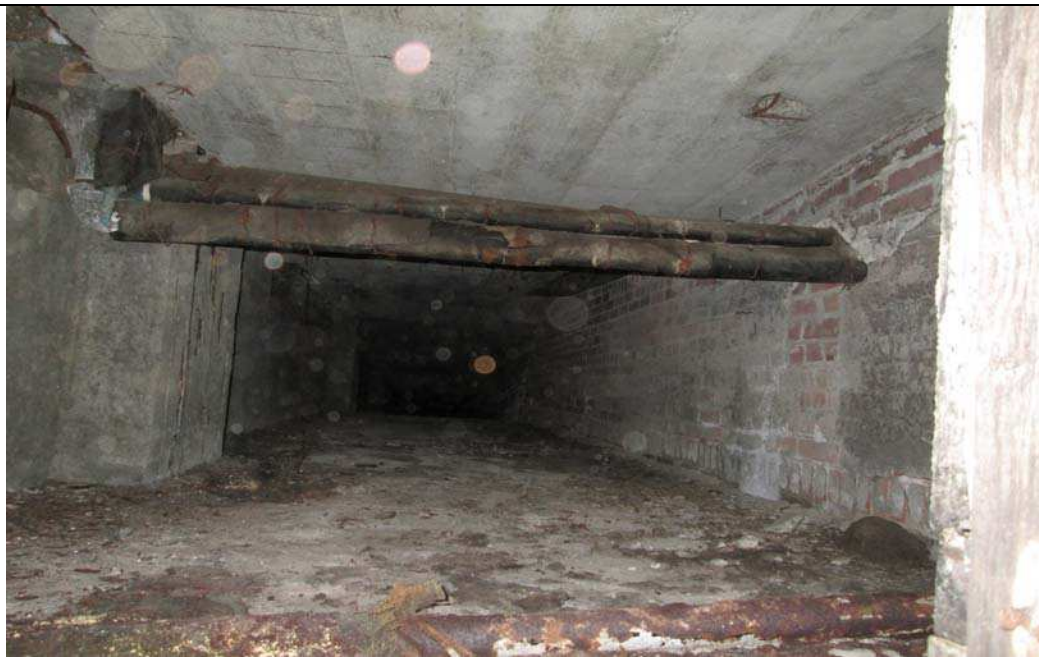
Photo 8 – View of Aircell Insulated Pipes in Basement Air Plenum
