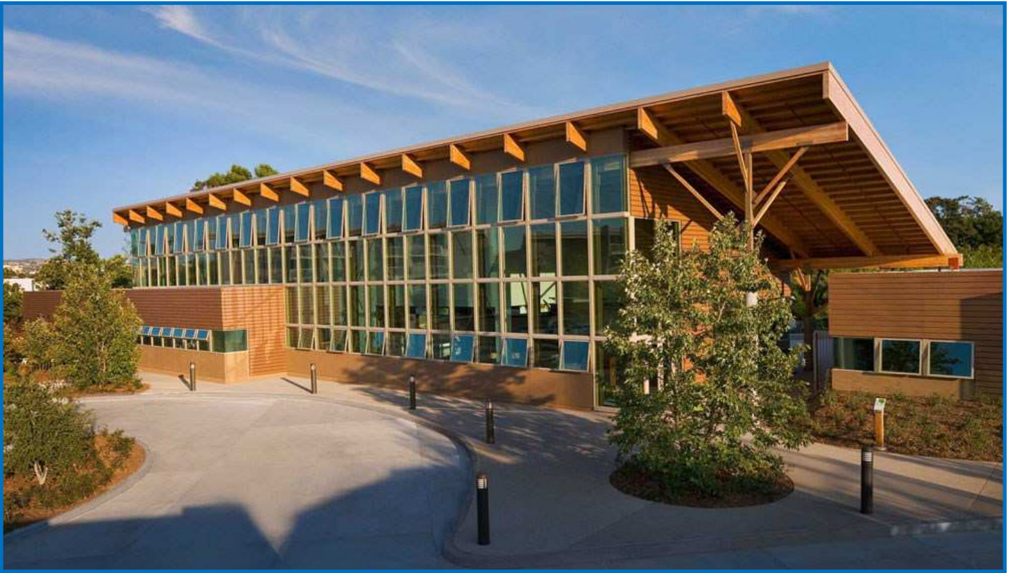
Figure 4-4: Example of a Nature Center using daylighting and natural ventilation to reduce energy costs; Environmental Nature Center, Newport Beach, CA.
