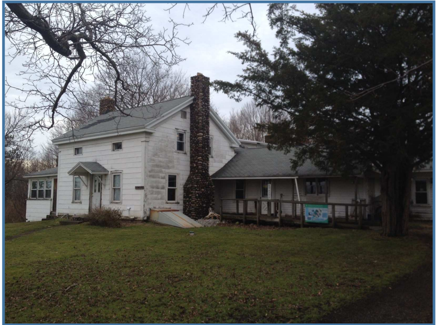
Figure 4-2: Jensvold Interpretive Building in January 2016; a roof patch is visible by the darker shingles located just below the left chimney. Photo courtesy of Cayuga County Planning.
