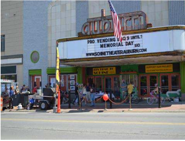
Existing Condition Photo of Façade Exterior
