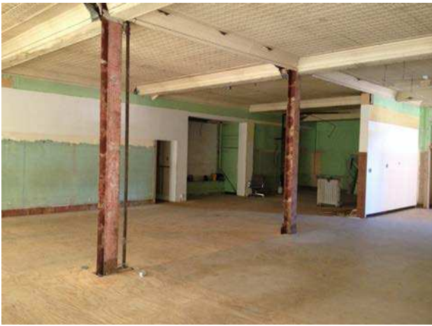
First Floor Existing Condition Image
