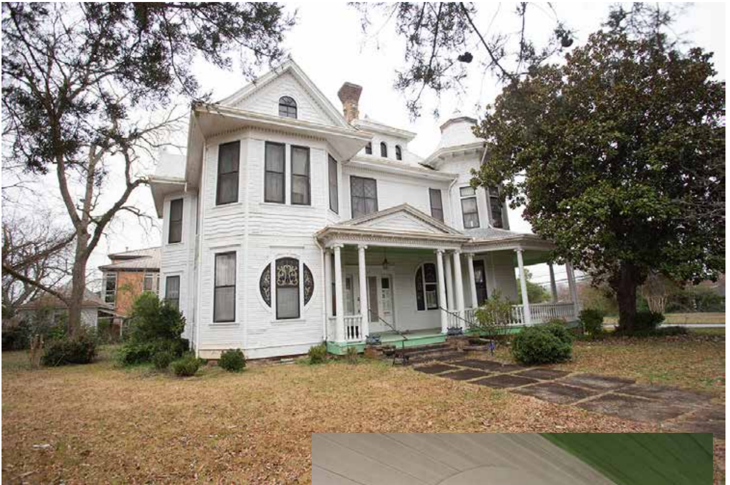
The Wren Home displays beauty and craftsmanship in its ornamented spire, ornate chimneys and unusual arched stained glass triple-windows.
