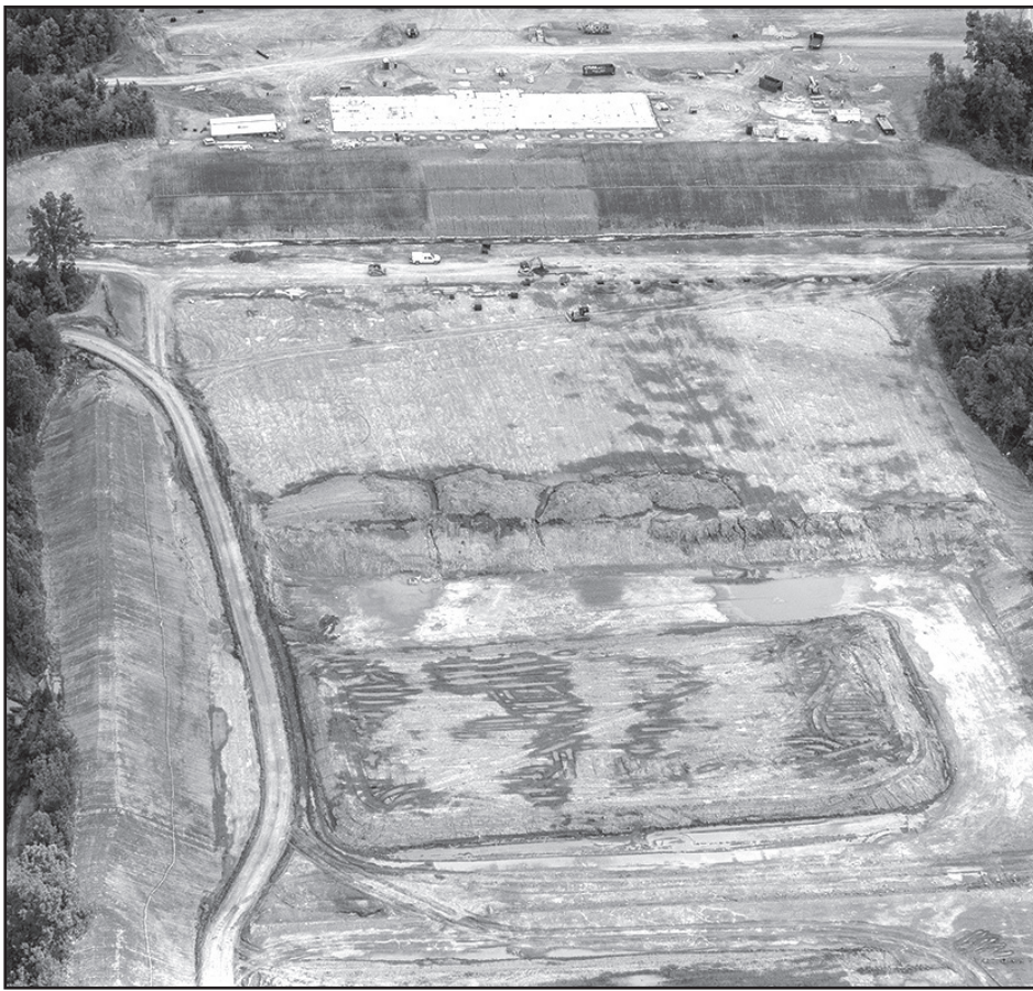
An aerial view of the $20 million marksmanship range under construction in Talladega County.
