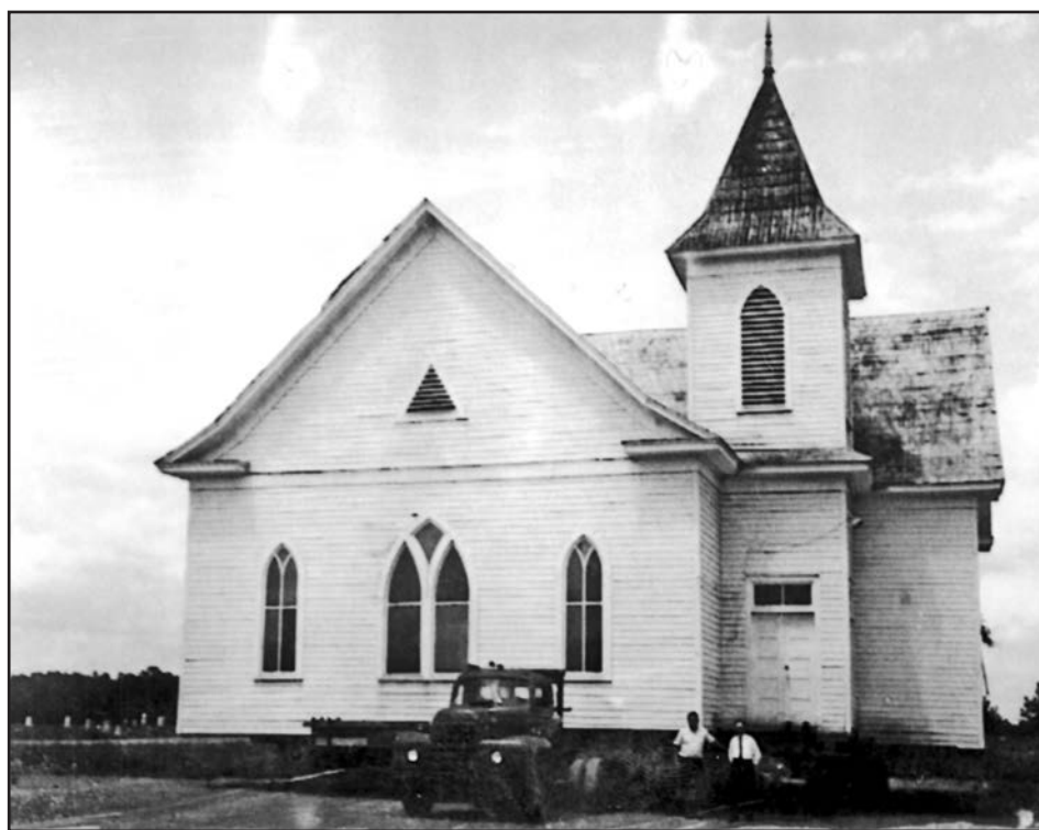
Coosa Valley Baptist Church had to be relocated for the dam construction. Workers managed to load the church onto a series of beams to relocate the building.
