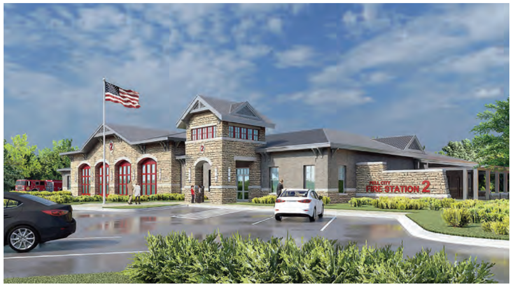
The new Pell City Fire Station No. 2.
