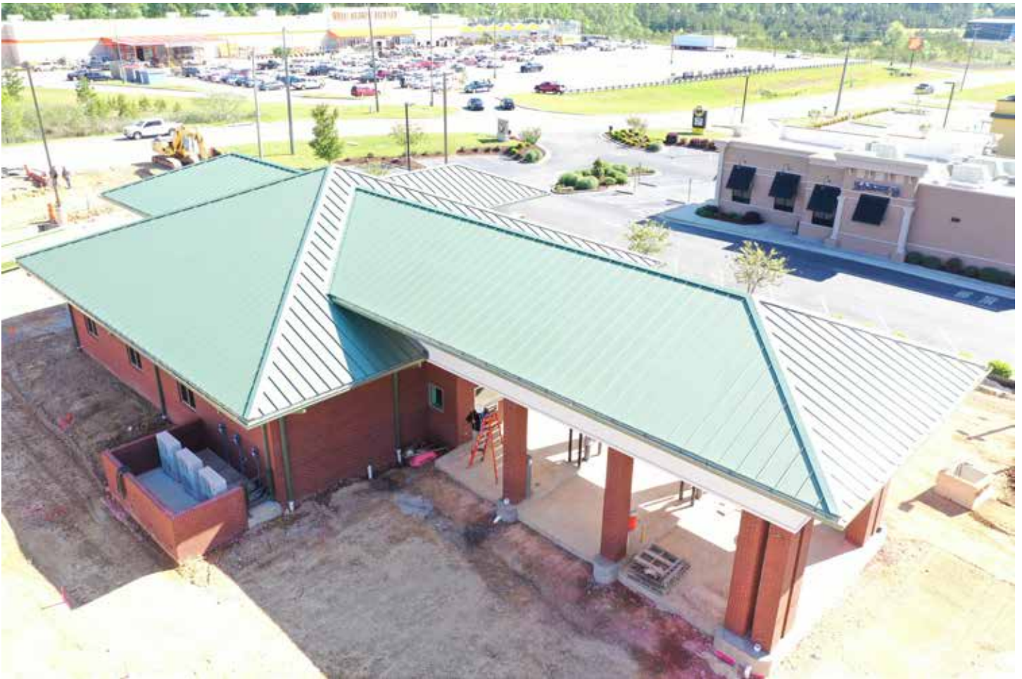
Construction began late last year at AOD's new office in Pell City, and plans are now underway for grand opening ceremonies at the Vaughan Lane location.
