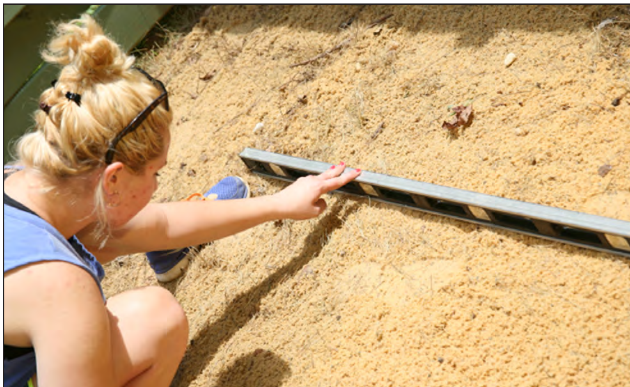
Hathorn checks the levelness of the area for her do-it-yourself patio project. "Making something look pretty and personal is fun," the teen-age blogger and home improvement enthusiast said.
