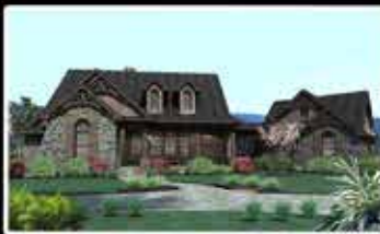
THE COTTAGE HOUSE
