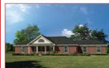
JASPER BRICK $124,900 3 Bedrooms, 2 Baths 2,294 Square Feet Under Roof
