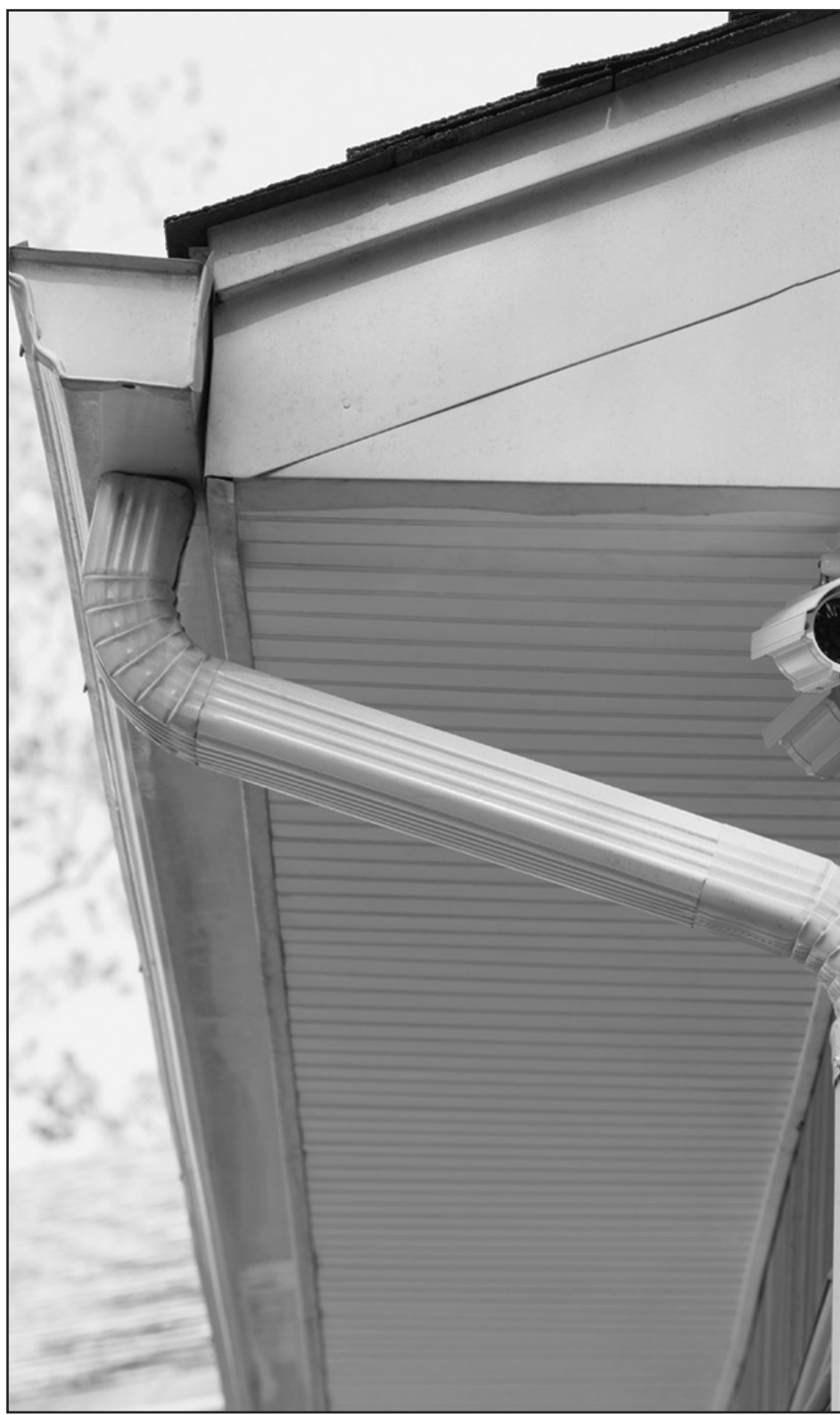
Each spring, homeowners should inspect their gutters to ensure the gutters are still attached to their homes and free of debris.
