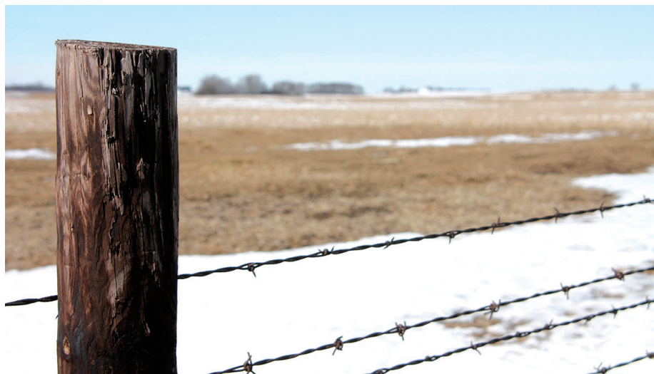
Barbed wire fencing, left unmaintained, can become dangerous to people and livestock. An expert shares tips for repair and replacement.
