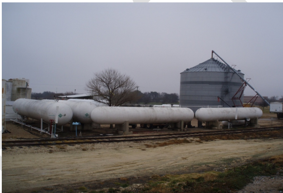
Figure 6. Anhydrous Ammonia Storage (Source: WFC Insurer)
