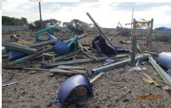
Figure 19. Damaged Playground Equipment (Source: ABS Consulting)
