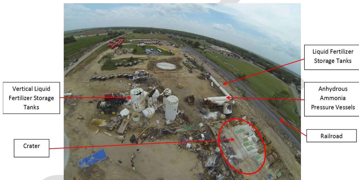
Figure 17. Anhydrous Ammonia Pressure Vessels (Source: CSB)
