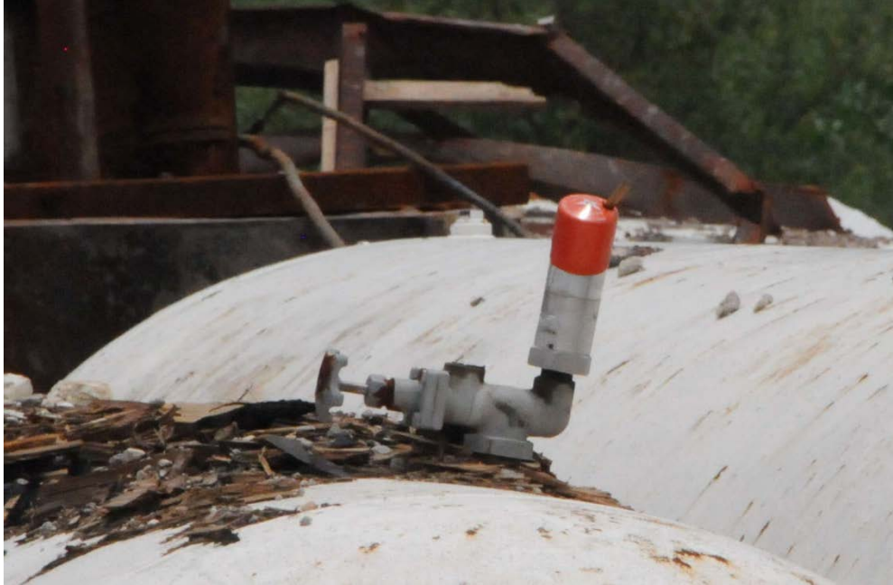
Figure 21. Anhydrous Ammonia Tank PRV, Post-Incident (Source: CSB)
