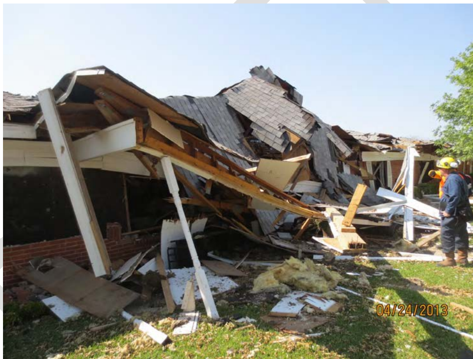
Figure 33. Damage to Reagan Street Entry of West Rest Haven (Source: ABS Consulting)
