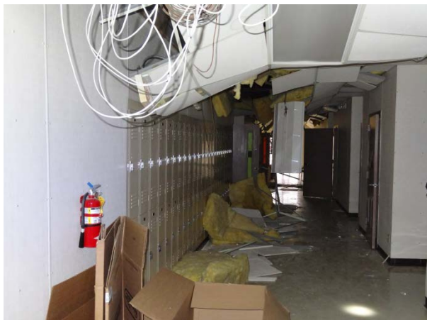
Figure 32. Classroom Annex Interior Hallway and Ceiling Damage at WMS (Source: ABS Consulting)
