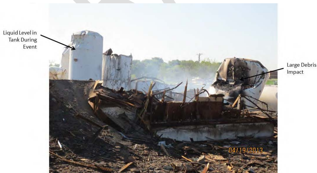
Figure 16. Liquid Fertilizer Tank Damage (Source: CSB)
