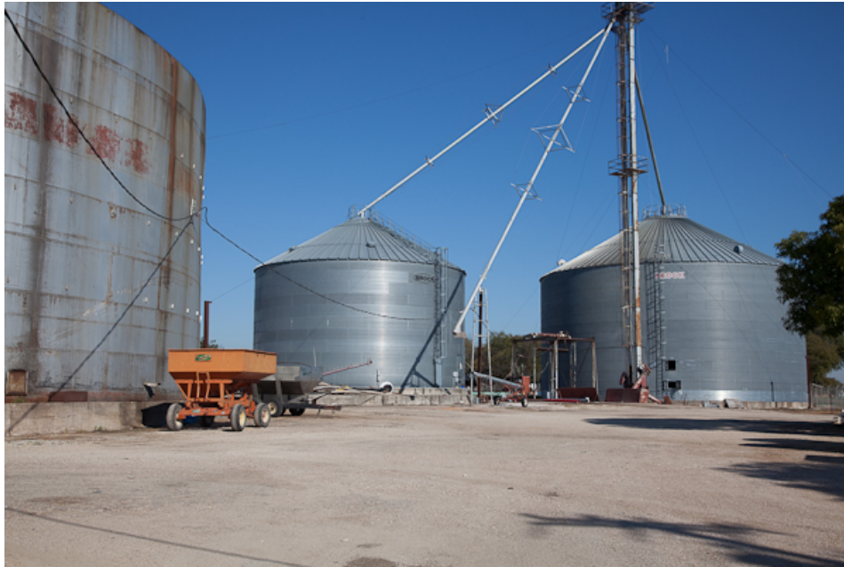
Figure 2. Grain Silos (Source: WFC Insurer)
