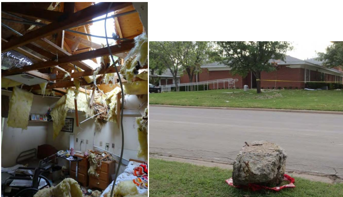
Figure 35. Crater and Debris (left) from Fragment (right) of WFC Facility Foundation that Impacted West Rest Haven (Source: ABS Consulting)
