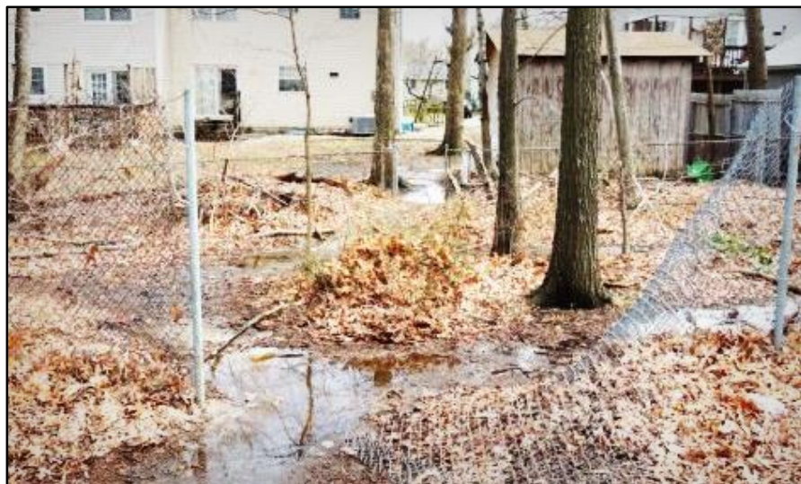
Figure 2: Inadequate perimeter fence.
