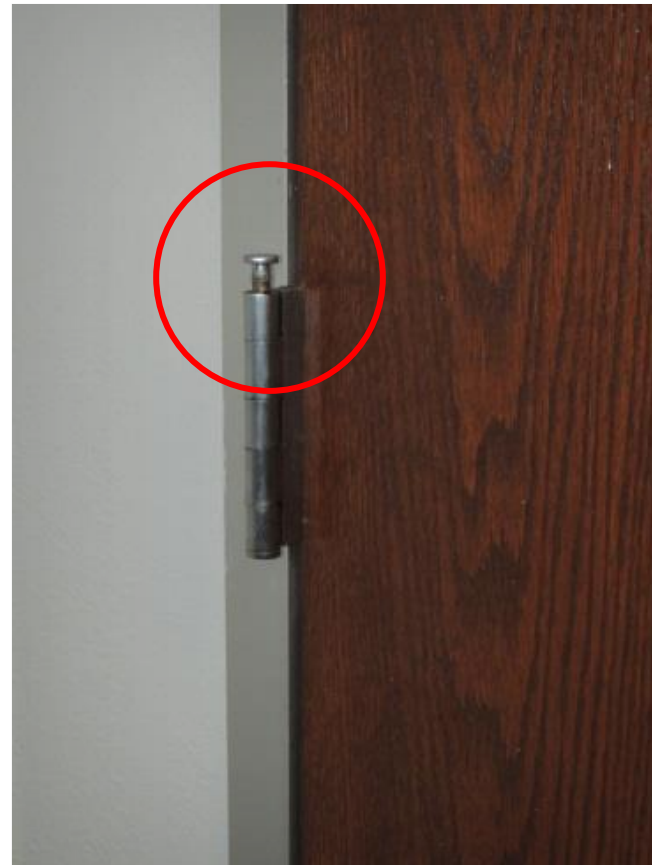
Hinges exposed to tampering
