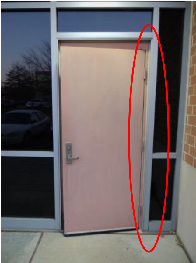
Hinges exposed to tampering
