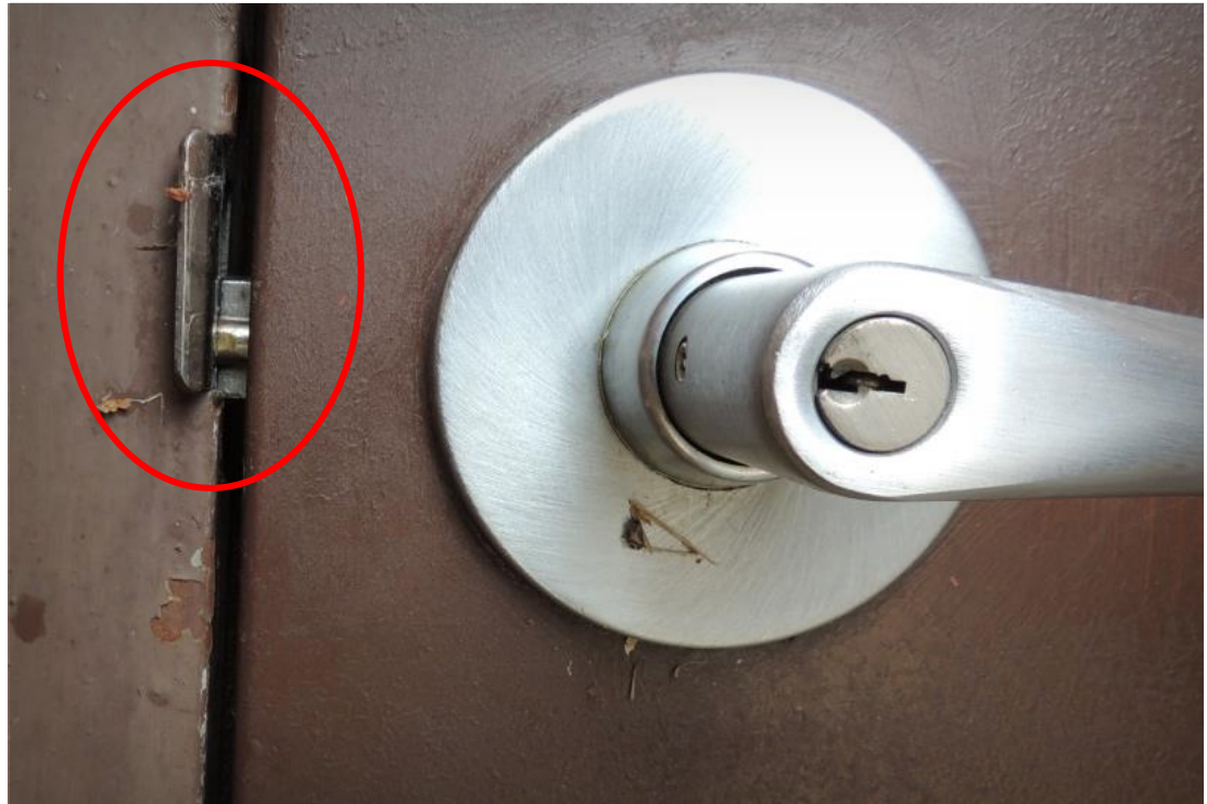
Exploitable to "carding"
