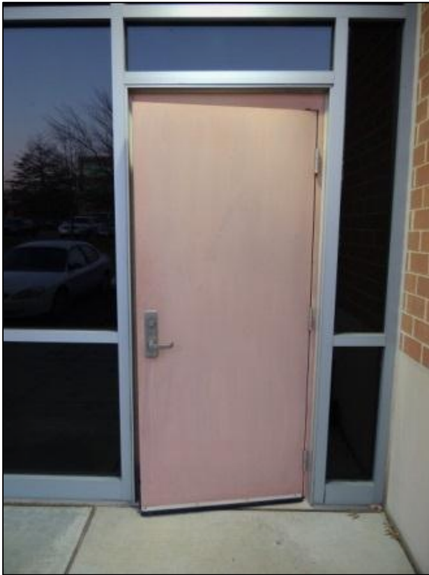
Figure 155: Unprotected hinges.
