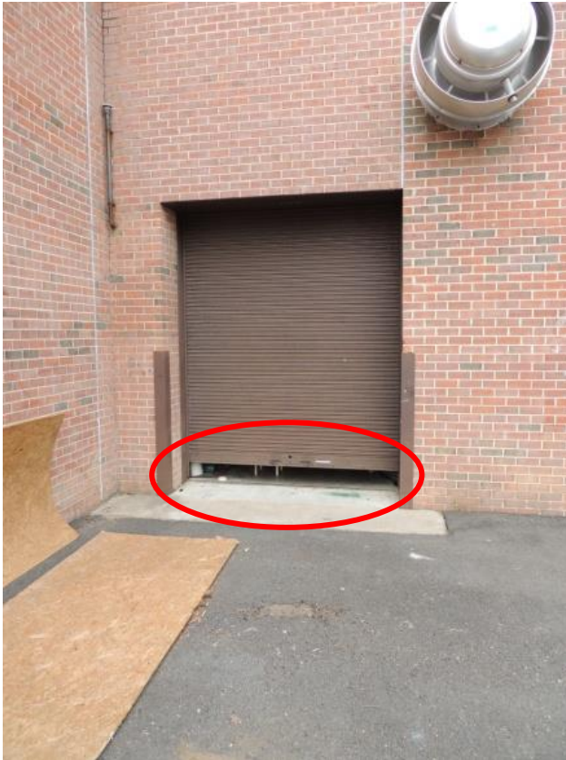
Unsecured service door
