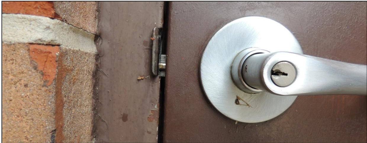
Figure 19: Exterior doors with locking mechanism on the outside of building.
