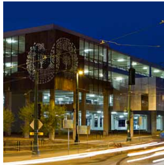
The Plaza Centro mixed-use development is an example of the Transit Oriented Development occurring in the downtown area.
