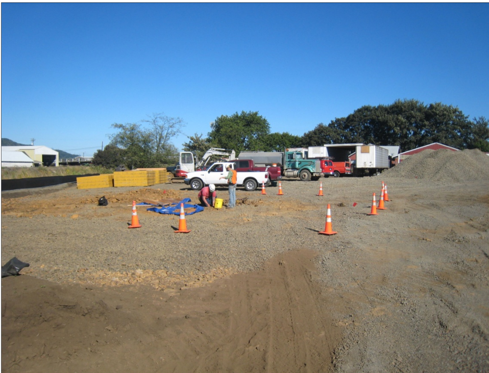
Figure 15. Overview of excavations in Area 3. Note the top of the red barn just visible at frame right, is also visible in Figure 5 prior to construction.
