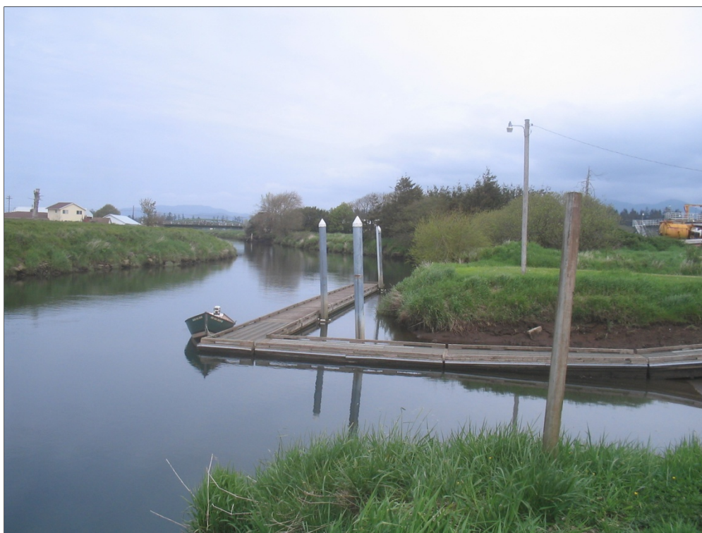
Figure 7. Overview of the site vicinity, facing north, showing the bend in the Trask River. The TWTP is just visible at frame right.
