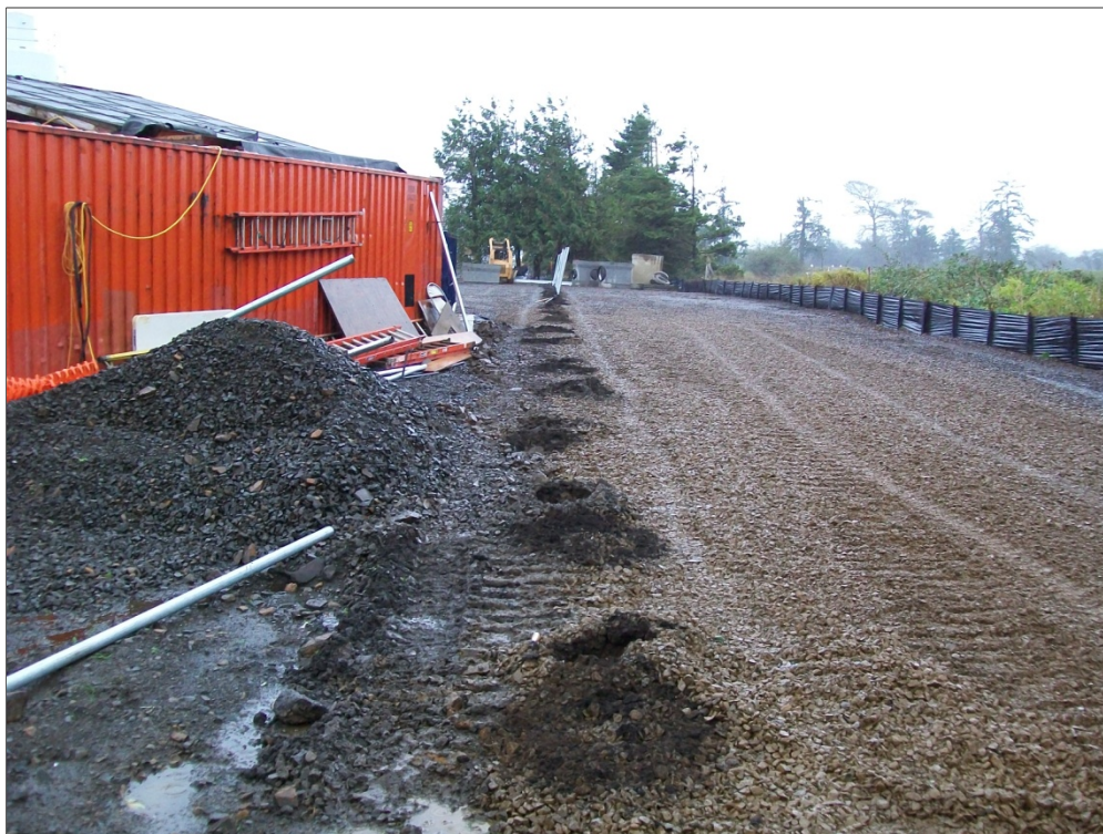
Figure 20. View of excavations for the installation of the security fence in the North Area.
