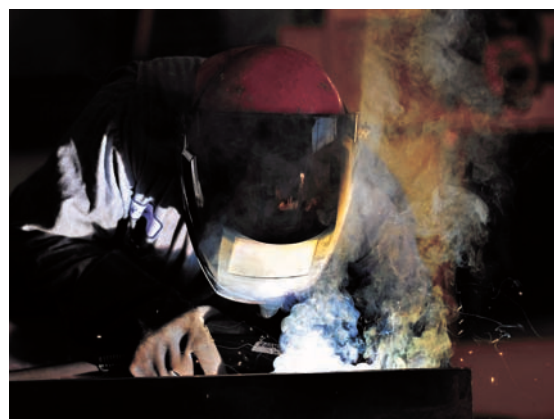
Ryan Whiteman welds metal brackets at American Bridge near Reedsport. The brackets are to be used in a building retrofit project the facility is working on.
