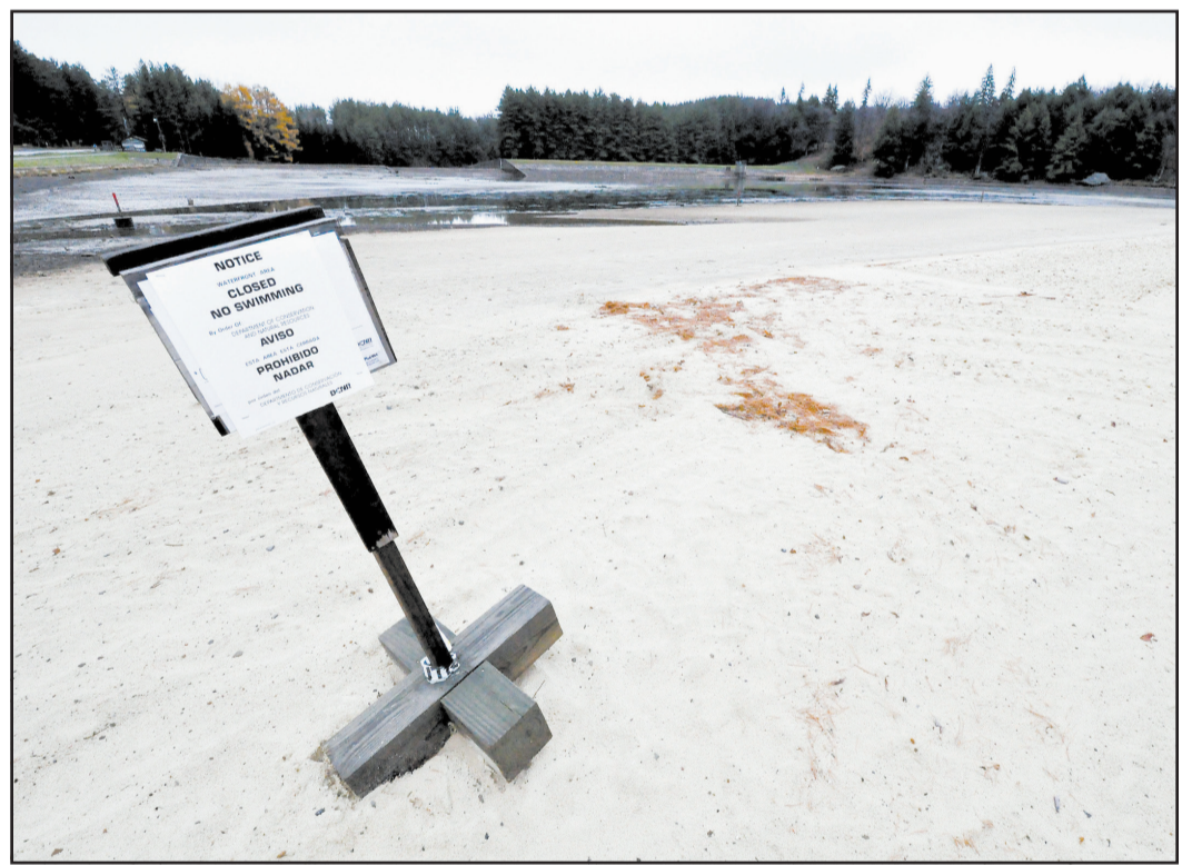
The state Department of Conservation & Natural Resources has performed a gradual five foot drawdown of Parker Lake to make repairs to an undermined concrete block wall adjacent to Parker Lake and Mud Run. The drawdown began Oct. 28. The lake will return to normal pool once the work is completed. (Photo by Katie Weidenboerner)
