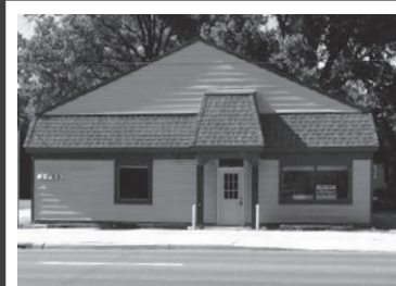
Commercial building, Rt 20 Saybrook. Just bring your business and move in. Call Ed Curie 223-1410
