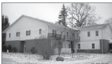
Rome. $235,000 Commercial unit w/13-2 bedroom apartments. Smoke detectors are monitored by Security Technologies. Some Refrigerators and stoves to remain. #3720261 Tara Dean 440-812-0508
