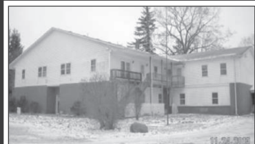
Rome. $235,000 Commercial unit with 13-2 bedroom apartments. Smoke detectors are monitored by Security Technologies. Some Refrigerators and stoves to remain. #3720261 Tara Dean 440-812-0508
