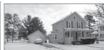
Jefferson. $89,500 3 Bdrm., 1 1/2 Ba. vinyl sided home w/beautiful deck. Lg kit. Beautiful oak trim throughout. New breaker box, updated wiring, plumbing, HWT, gas furnace and CA. Detached gar. w/vinyl siding and new metal roof. #3765308 Denny Ruck 440-812-5245
