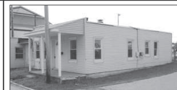
Jefferson Vlg. $30,000 Could be business and residential. 4 large rms, kitchen, bath, dining area. Newly painted, windows, separate entrances. #3743933 Carol Fulwiler 440-969-0674 Sean Kennedy 440-415-4090
