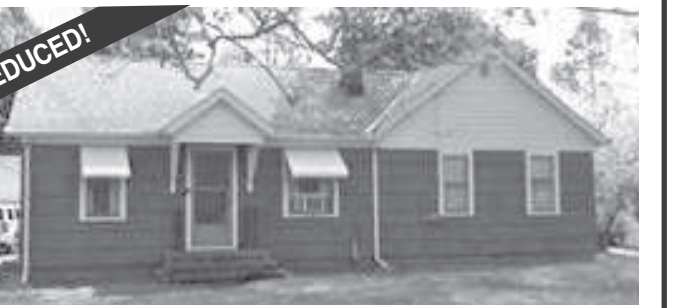
2172 S. Broadway-Geneva - Well maintained 3 bedroom country home with large barn with stalls and work area with electric, 2 car detached garage with new doors. on 3.46 acres. Living room with built in window seat. Eat-in country kitchen appliances stay refrigerator is 2 years old. Many updates including plumbing, electrical, newer roof, gutters, garage doors, newer water line. Gas line on property. Partially finished basement with fireplace, kitchen area, full bath. Close to covered bridges, wineries, shopping, Spire Institute, I-90 and metro parks. Home warranty included. $125,500 Sherri Jastrzembki 440-415-2026
