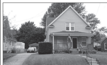
Conneaut $84,900 Lovely Colonial home redone from top to bottom. 3BR/ 2 BA with lg rooms. 1 car garage and above ground pool. #3736289 Lois Blank 440-265-0820
