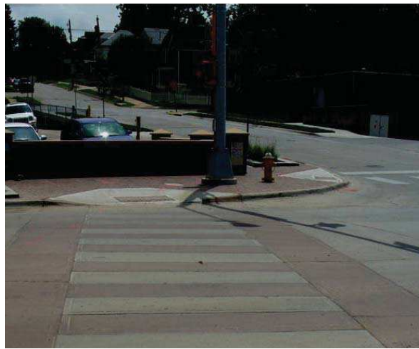
Color Concrete Crosswalks
