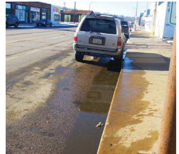
Ponding Water Along West 7 th Street
