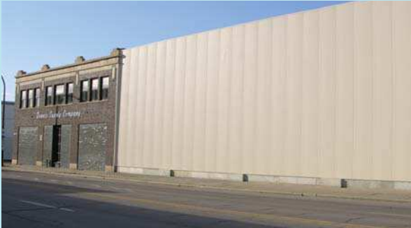
Dennis Supply Building - Existing Facade
