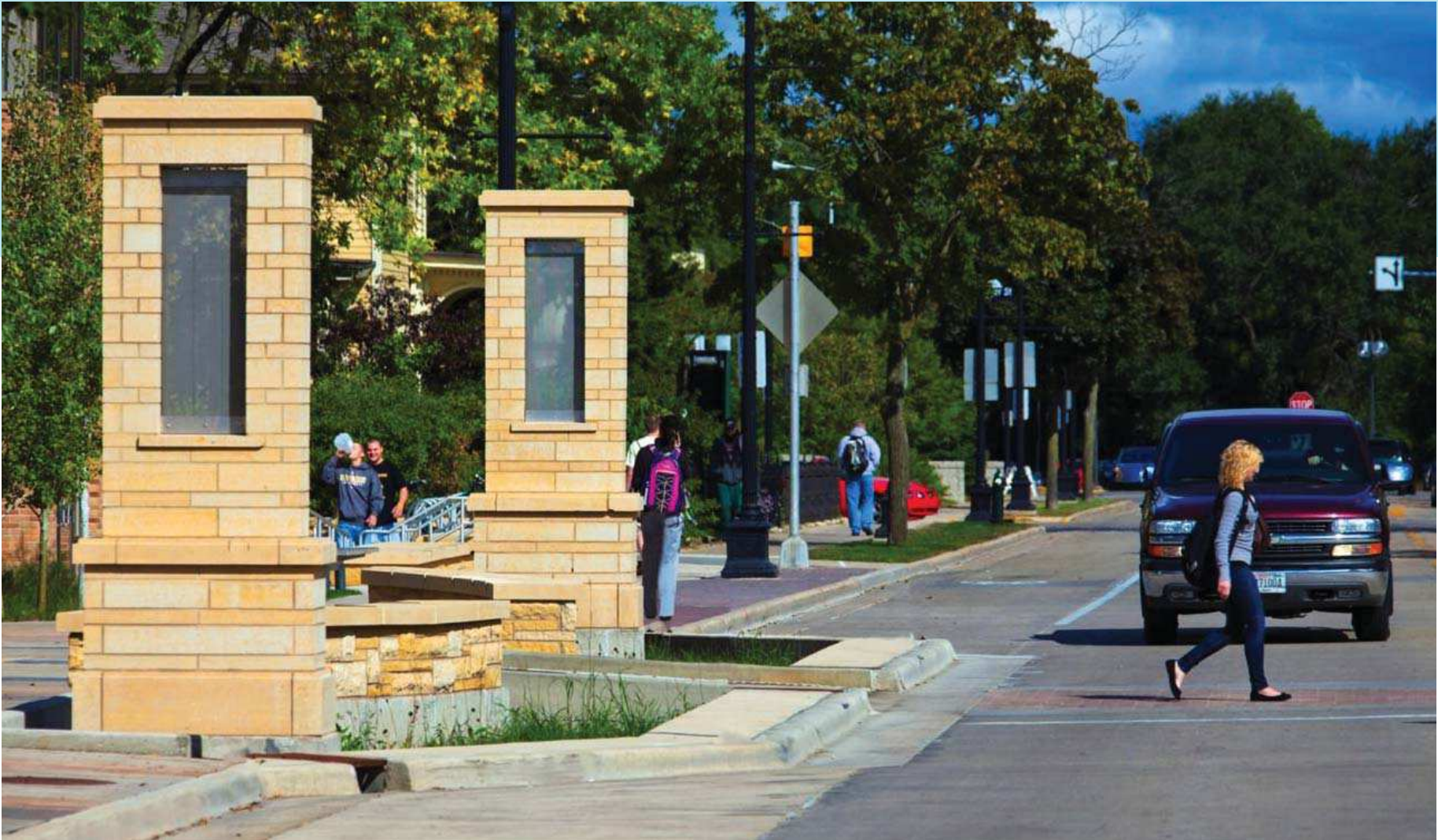
Rainwater planters similar to these would clean storm water before it is released into nearby Perry Creek.
