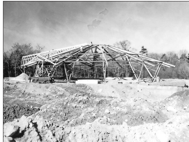
The theater under construction in 1955.
