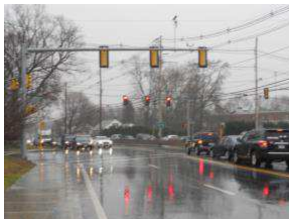
Left turn lane at Liberty Street aligns with through lane on departure side
