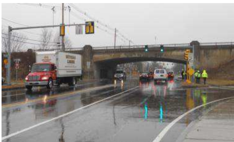
Route 62 westbound at Route 128 northbound ramps
