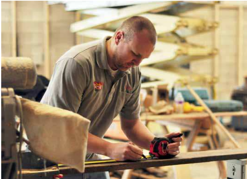
Billy Stronks, co-owner of Teton Fitness, spends another afternoon working on the construction of the new gym in Ashton. Photo by Heather Randall
