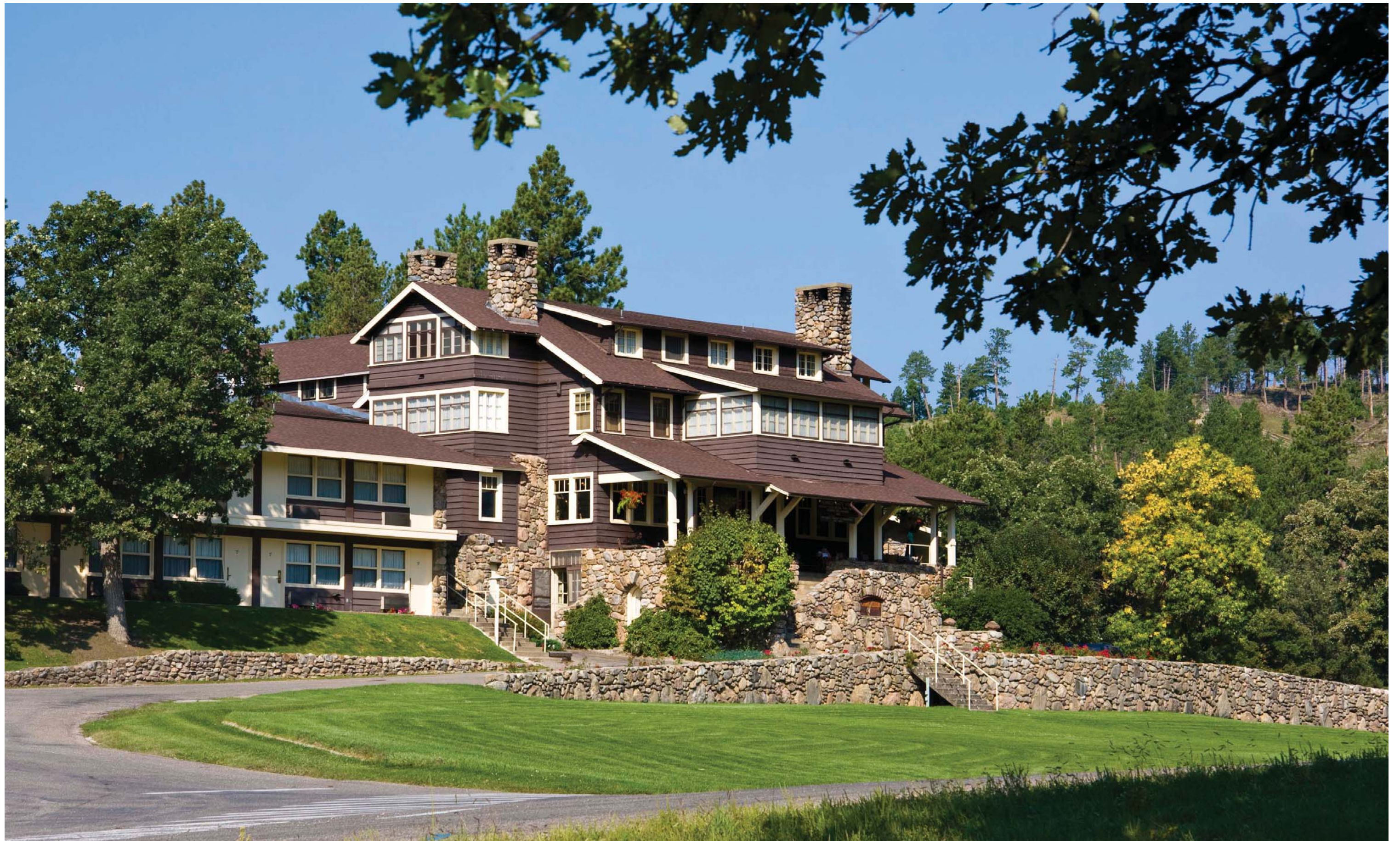
RENOVATE THE ORIGINAL ENTRANCE FACADE (STEPS, ROCKWORK, SIDEWALK, RETAINING WALLS) AND REPLACE SIDING AND WALLS.
