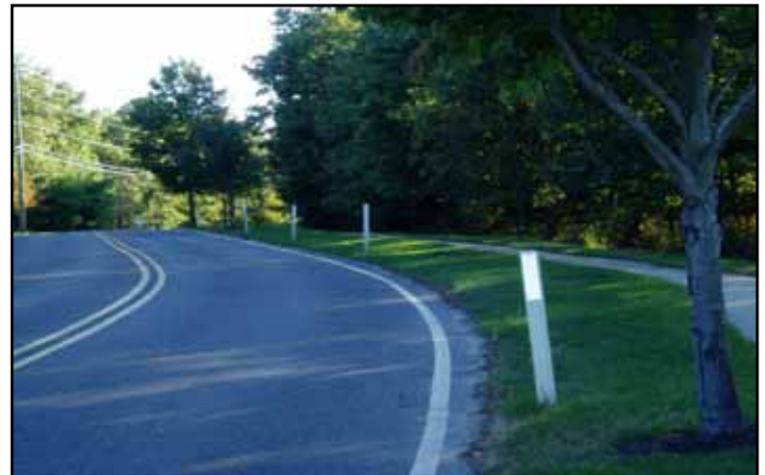
Extra reflective posts have been installed.
