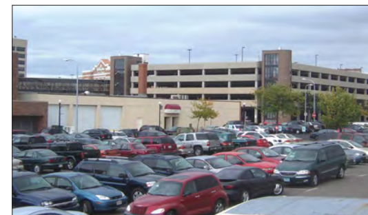
La Crosse Center Parking Ramp, La Crosse, WI C.D. Smith provided General Contracting services for a two-story addition to the La Crosse Center parking ramp.
