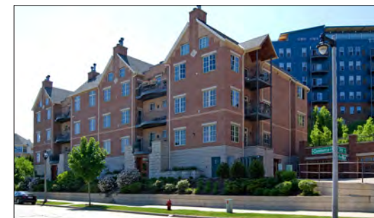
Commerce Bluff 130,000 sf mixed-use, multi-phase development overlooking the Milwaukee River including condominiums, offices, and European-style cafe. Architecture by TKWA.
