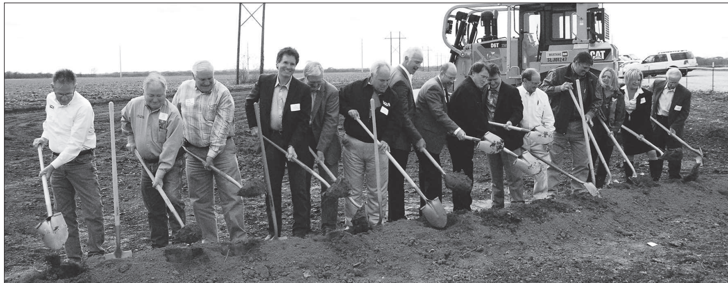
Key stakeholders join the Lower Colorado River Authority in breaking ground in December at the site of the Lane City Reservoir. Wharton Journal-Spectator file photo
