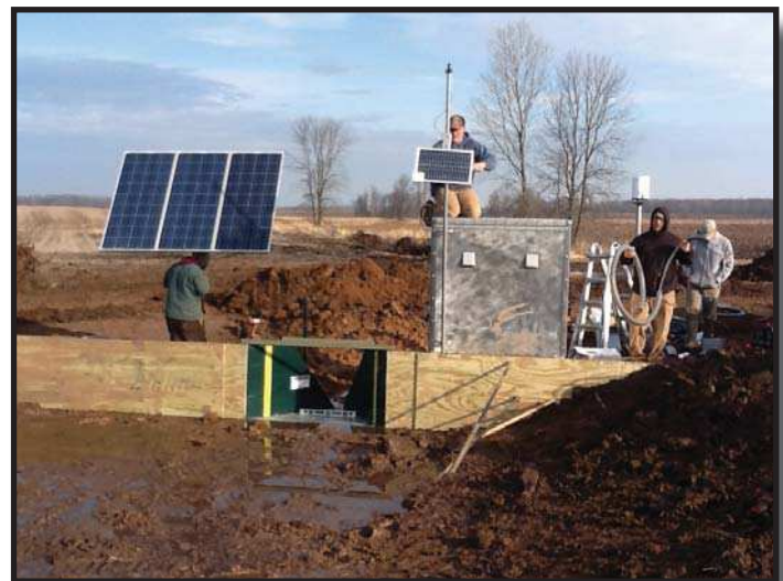
Edge of field monitoring equipment being installed on agricultural land in a Phosphorus Reduction Priority Watershed.
