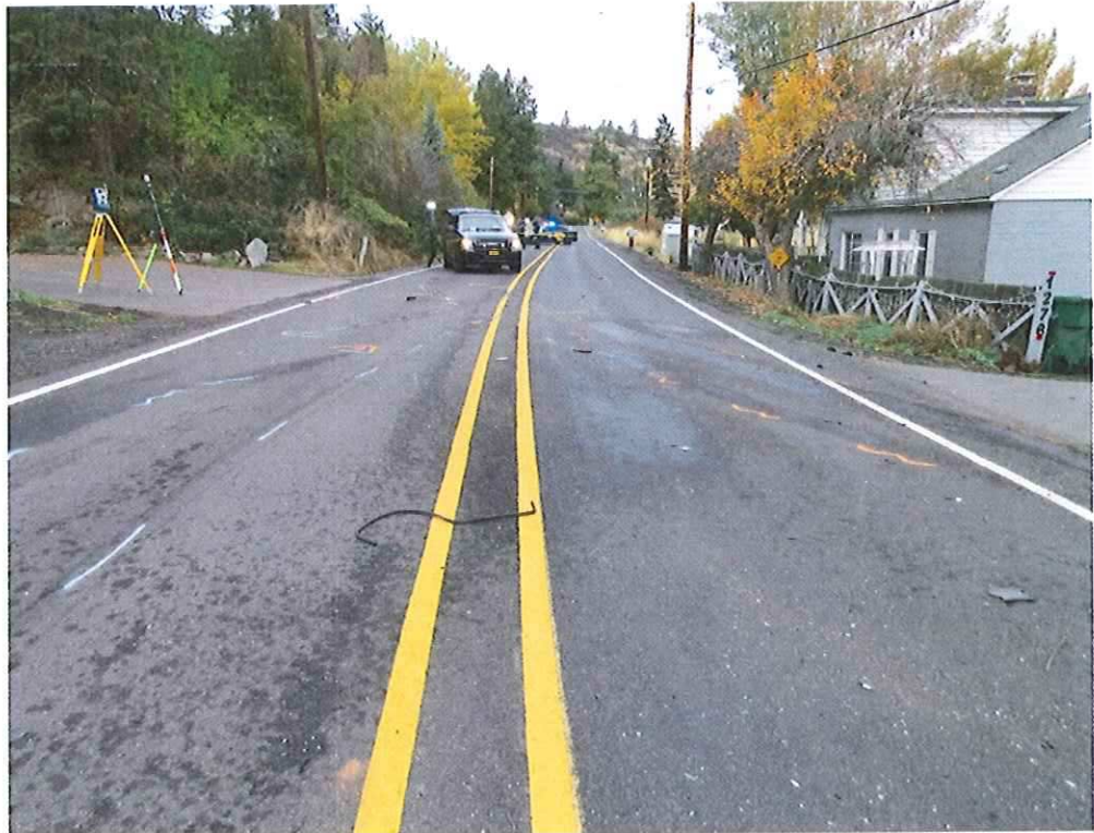
Photograph 4624 – Lakeshore Drive looking westbound.
