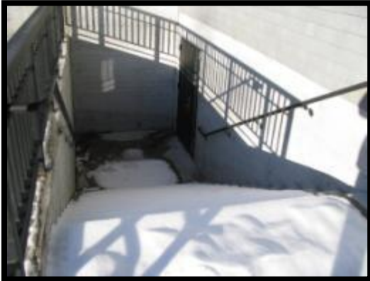
Basement entrance on west side addition
