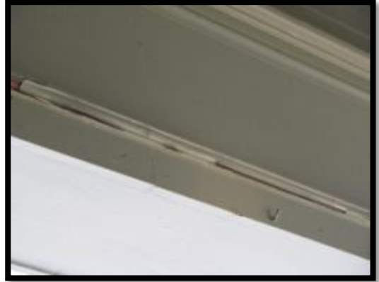
Porch Ceiling on Story Mansion
