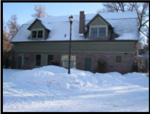
View of carriage house from north
