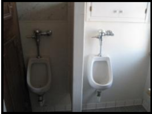
Second Floor Bathroom
