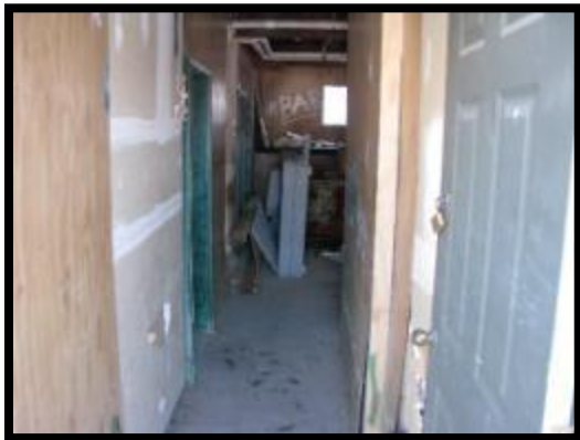
Carriage House Entry
