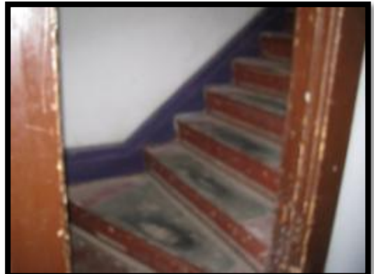
Stairway to Third Floor
