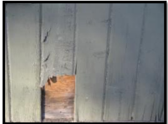
Exterior Wall on Carriage House
