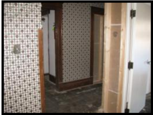
Second Floor Landing
