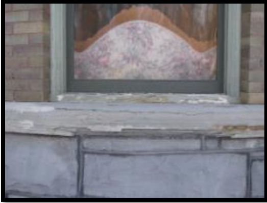
Window Sill on front of Story Mansion
