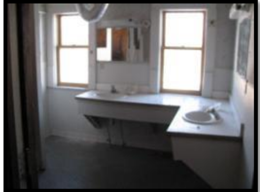
Second Floor Bathroom
