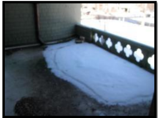
View of Second Floor Balcony from Study
