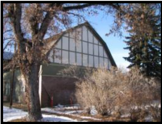
View of carriage house from southeast
