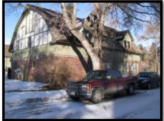
View of carriage house from southwest
