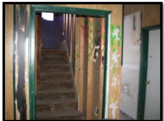
Stairway to Carriage House Loft
