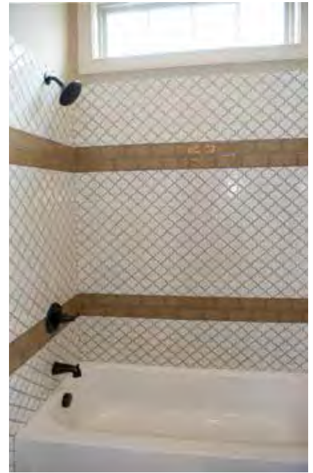
↑ A simple tile set on point and grouted in the shade of the accent ribbons makes a big impact in a small space.
