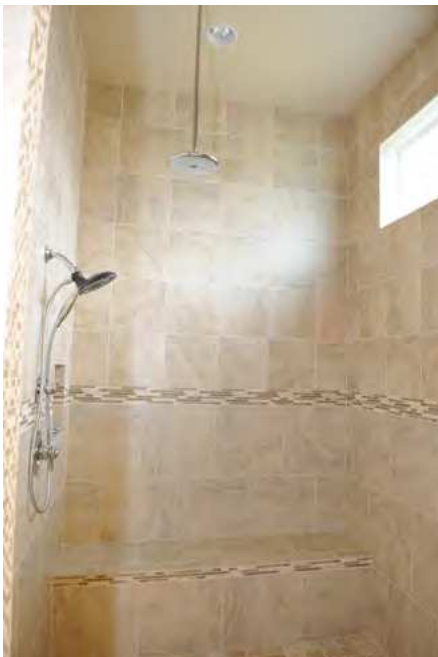
↑ A pair of showerheads includes a wall mounted unit and a rain unit that the homeowner is really glad to have included in the design.
