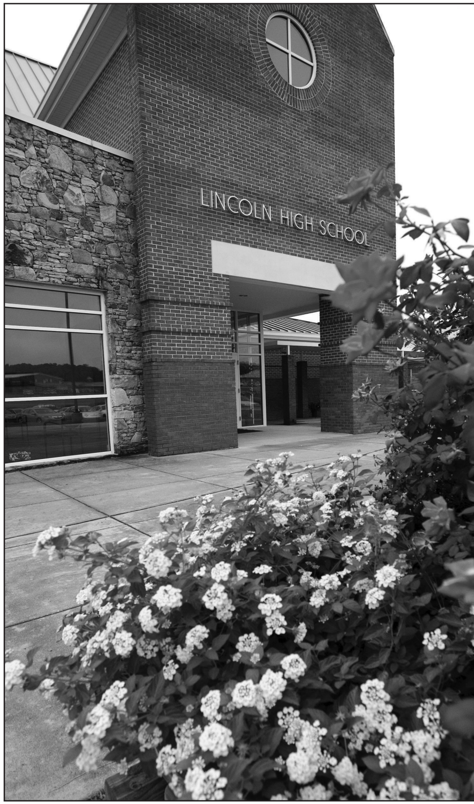
Lincoln High School was among the Talladega County schools that implemented the new technology initiatives in January.
